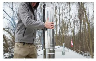
Connect the 2<sup>nd</sup> insulated chimney piece onto the first.
