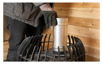
Place the shorter chimney connector piece onto the flange off the heater.
