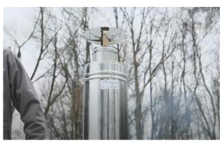
Slide the chimney cap into the top stack and fold over the tab to secure it in place.
