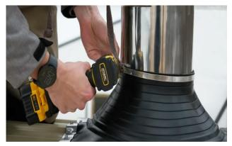
Place the hose clamp over the membrane and tighten the screw.
