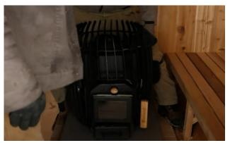
Bring the heater in and place it on top of the floor shield.
