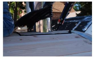
Lift the membrane out of the way and apply the included roof sealant on the inside of the outline.
