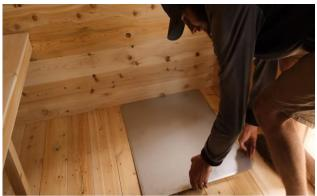
Place the heat shield on the floor in the sauna where the stove will be.
