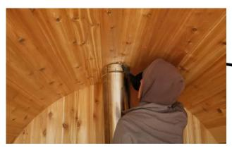
Use the chimney stack to trace out a circle around the marks made in the previous step.
