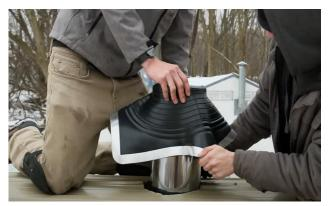
On the top of the sauna, slide the rubber membrane over the chimney stack.
