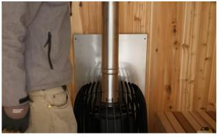
Place the longer chimney connector piece onto the short piece.
