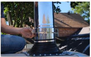
Attach the support strap around the chimney pipes and tighten up.
