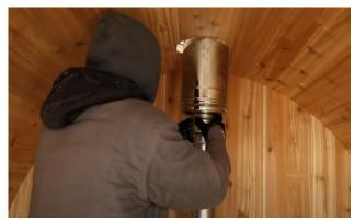
Slide the bottom chimney stack through the roof hole and into the connector pipe.
