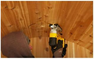
Cut out the circle with a jig saw.
