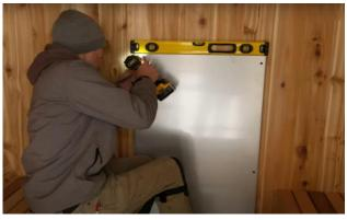
Ensure the heat shield is level and attach to the wall with  $1 \frac{1}{2}$ " (38mm) screws.
