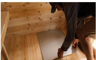
Place the heat shield on the floor in the sauna where the stove will be.
