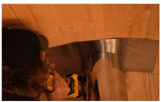
Install the 2 halves of the chimney hole shield around the chimney on the inside to cover the hole and secure with  $6 - 1 \frac{1}{2}$ " (38mm) screws.
