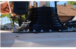
Slide the membrane back down and secure using the included self-sealing roofing screws every 1-2" (25mm to (51mm)
