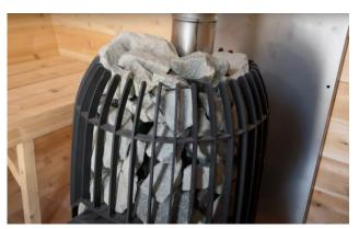
Place the rocks in the heater until they are 2" (51mm) above the top of the heater.
