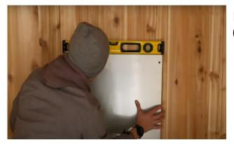
Place the wall heat shield so the bottom is around 2" (51mm) from the floor of the sauna.
